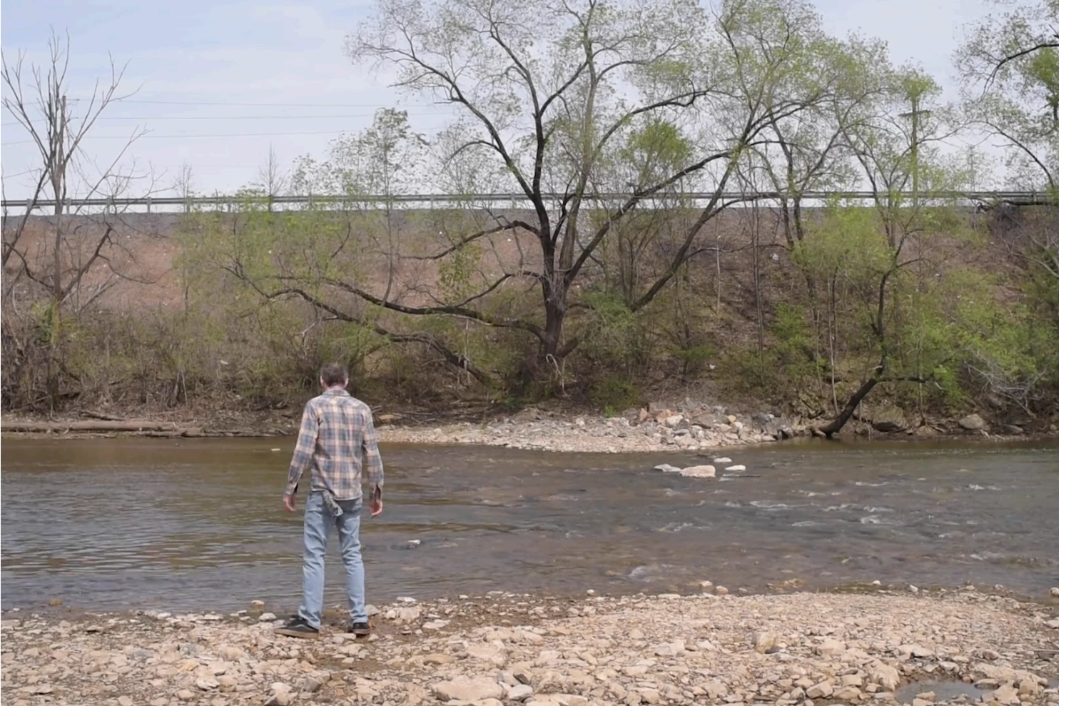
Rubble remaining from the Bedford dam removal; Mr. Fetterman at the now undammed river. Andrew Mangum for The New York Times
